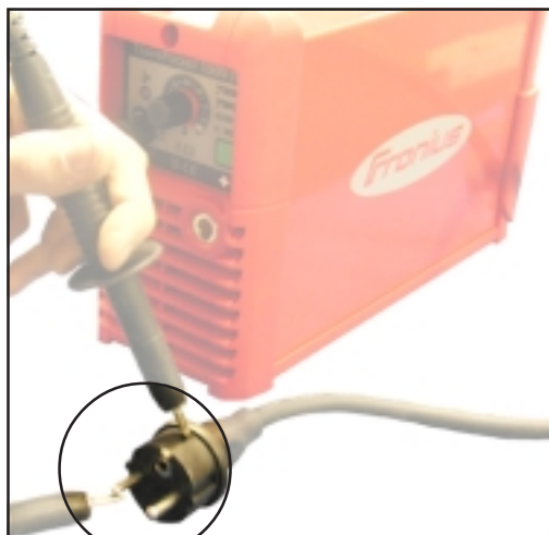
Fig. 24 Insulation test - Primary circuit / earth
