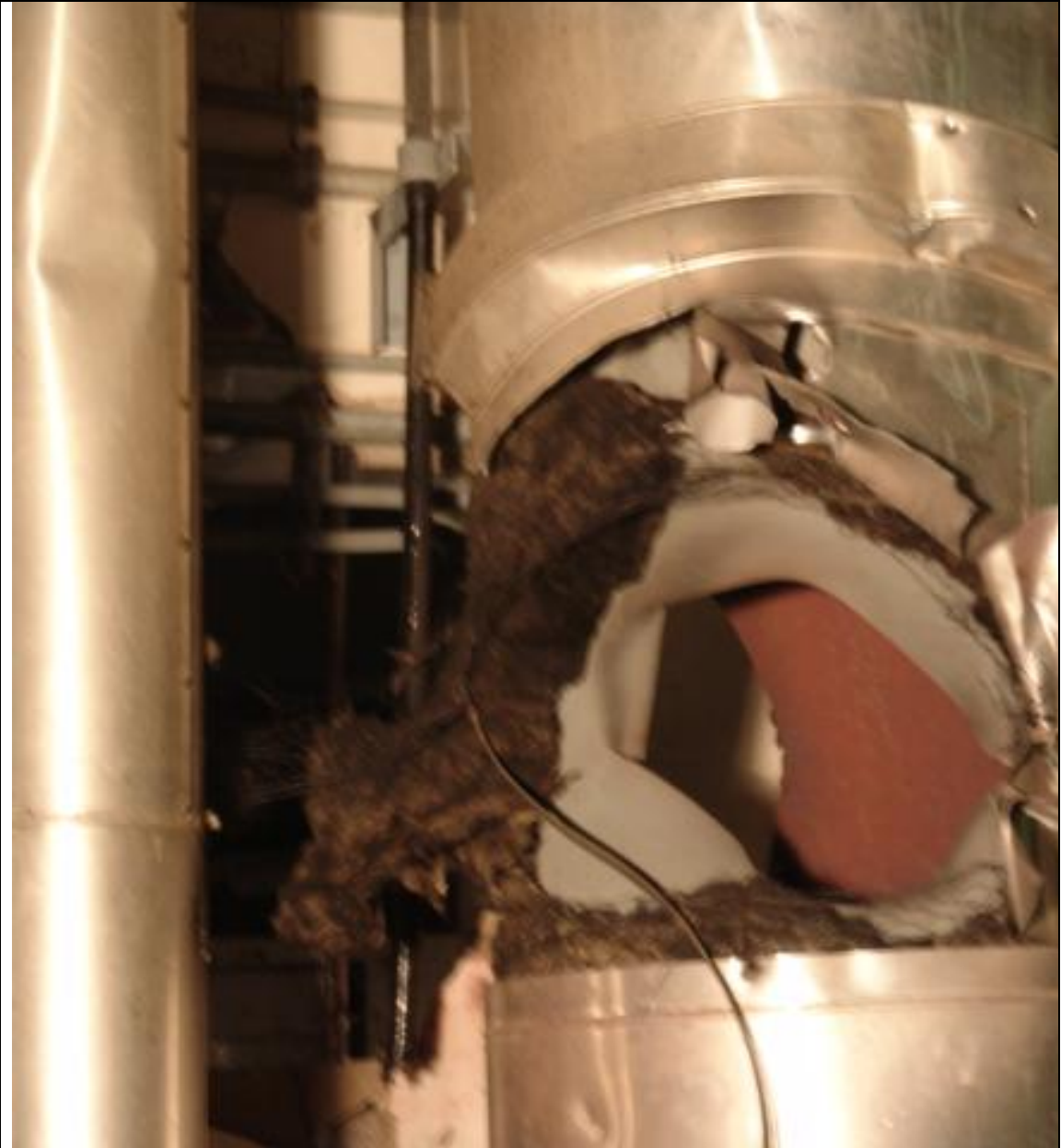
Pic# 10: Flying Piece Damaged LP Steam Line to Dearator.
