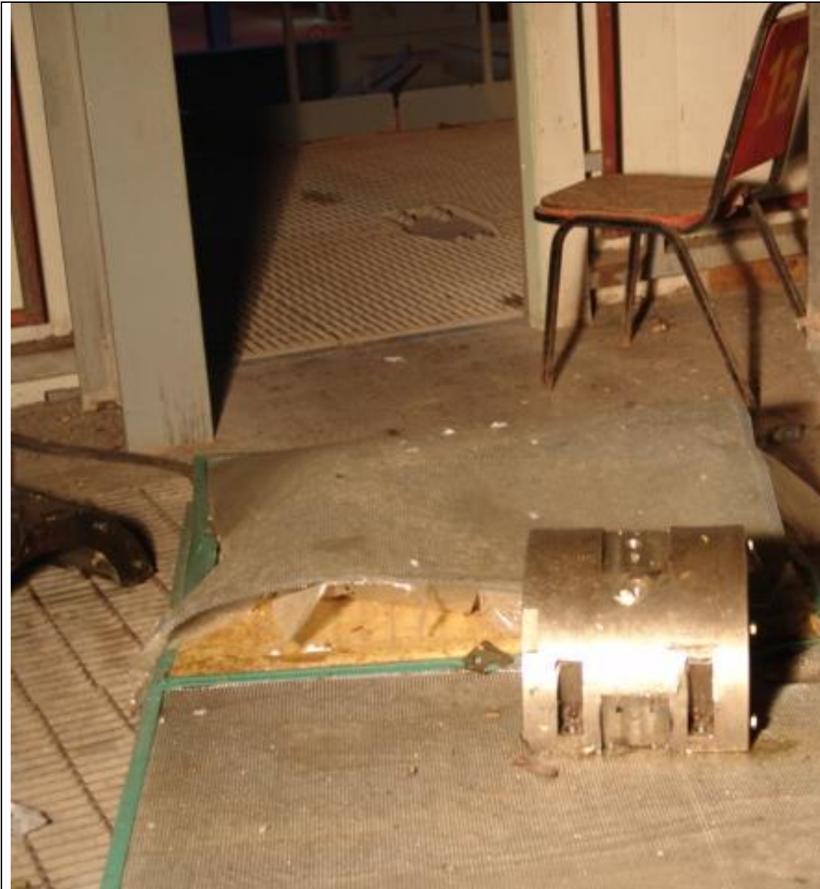
Pic# 7: Turbine Generator Bearing Lying Near Door on Desal Side.
