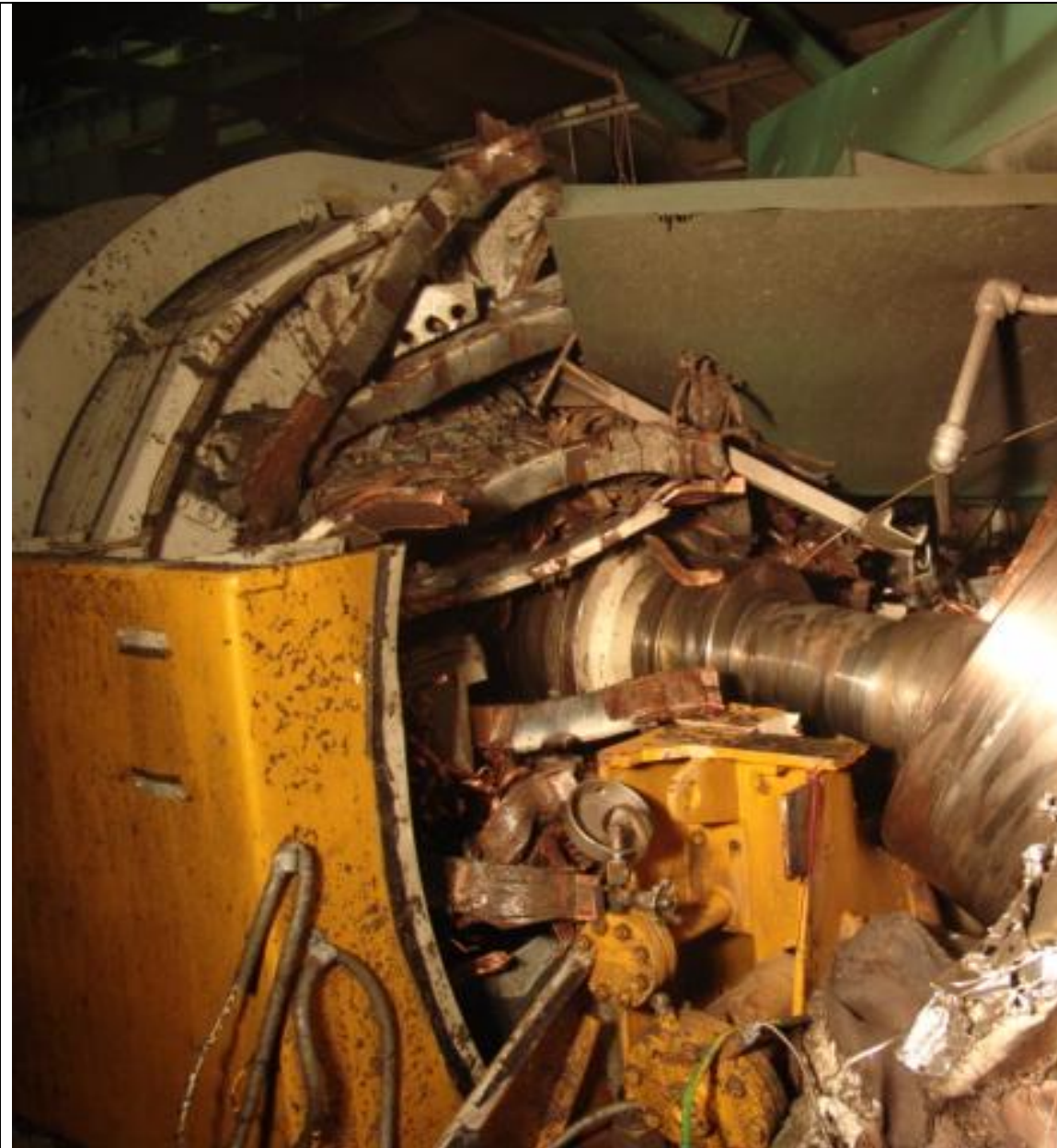
Pic# 9: Damage to Generator on Turbine Side-Retaining Ring Flown out towards Turbine Side.
