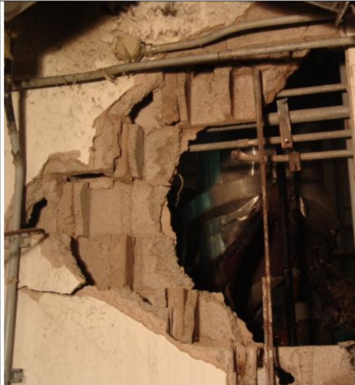
Pic# 17: Damage Occurred to Switchgear Room Wall –Viewed from Switchgear Room.
