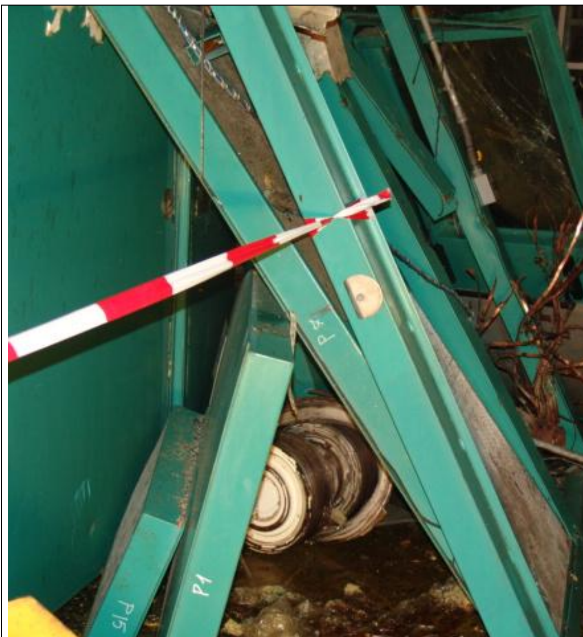
Pic#14: Sheared off Part of Generator Rotor Shaft of Exciter end.
