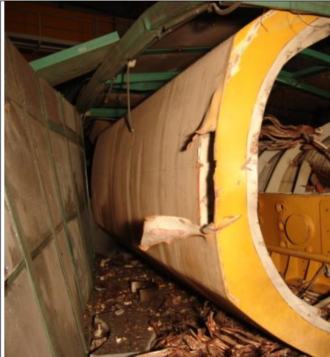
Pic# 4: General View of the Generator Viewed from Exciter Side.
