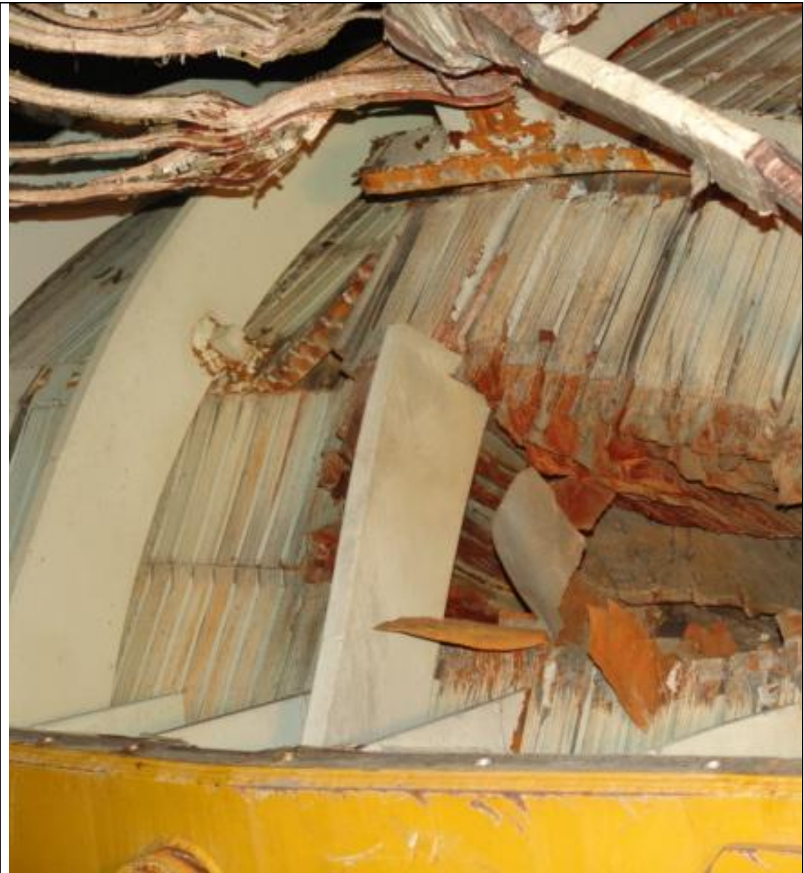
Pic# 16: Damage to Generator Stator Core.
