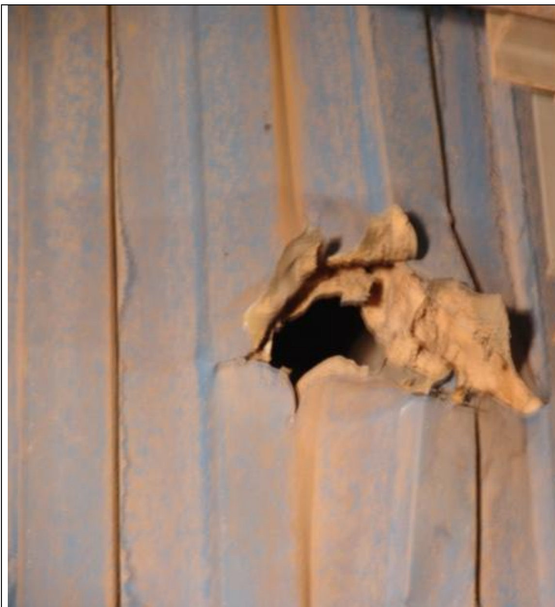
Pic# 12: Damage to Side Wall between Switchgear Room and Boiler
