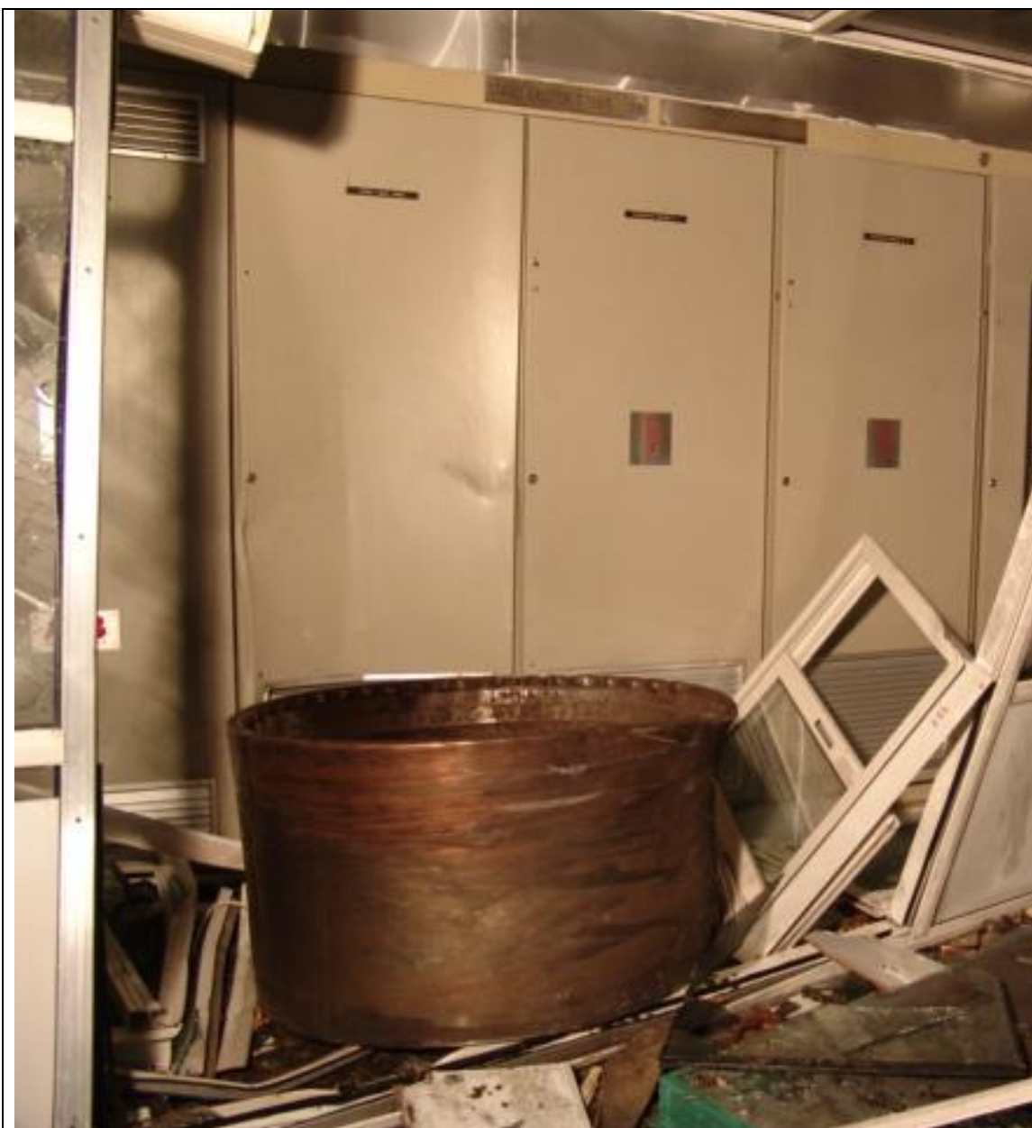
Pic#5: Exciter End Generator Rotor Retaining Ring Lying Near Static Exciter Panel.
