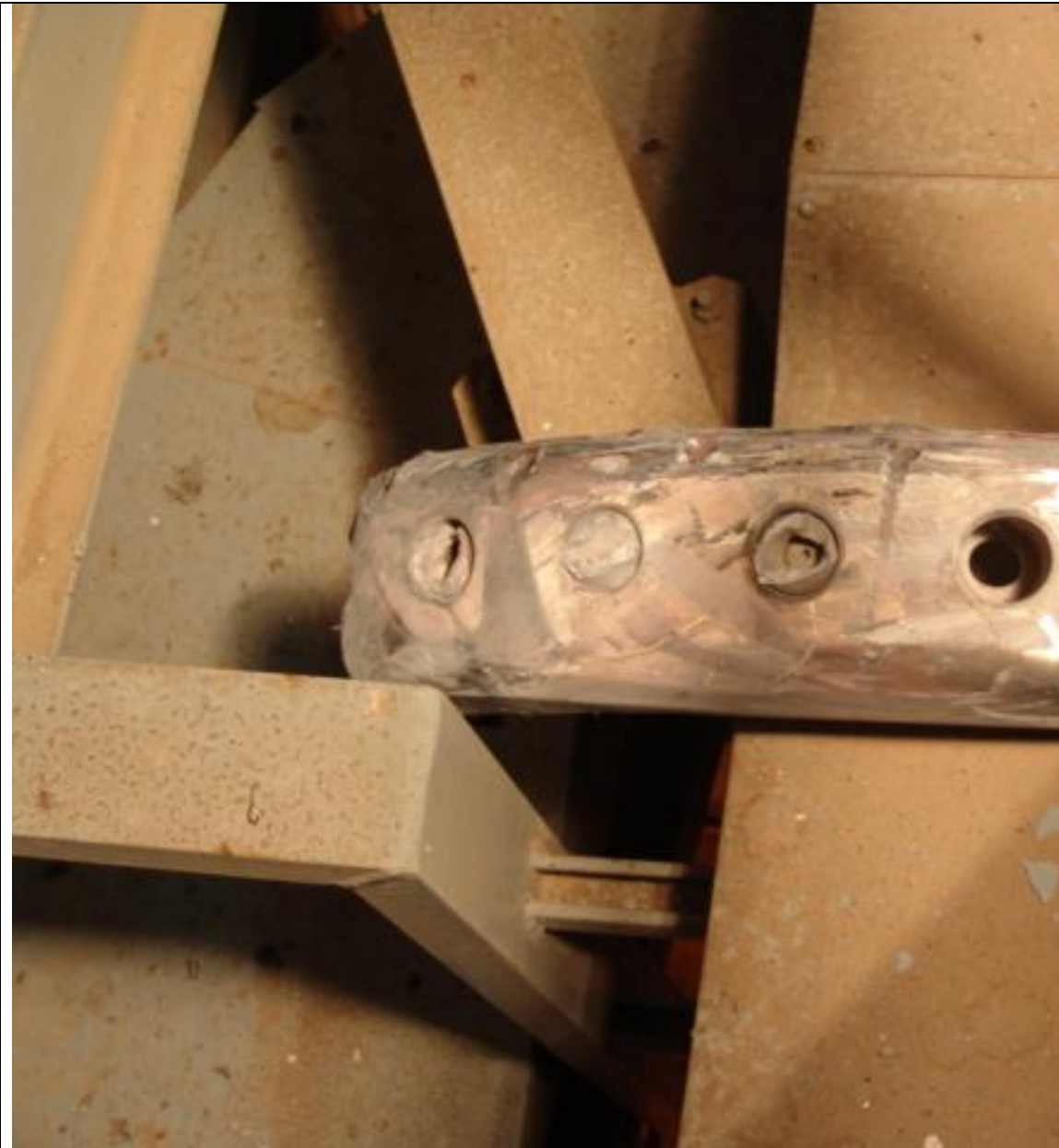
Pic#13: A Piece of Generator Flown to Boiler Area After Piercing the LP Steam Pipe, Switchgear room walls and one I- beam.
