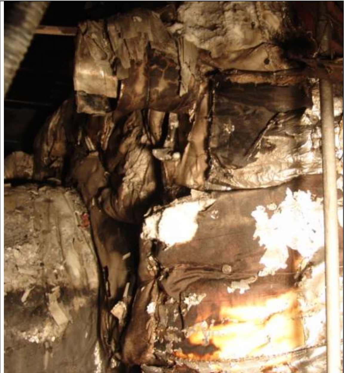
Pic # 8: Damage to Turbine Insulation- HP Side.
