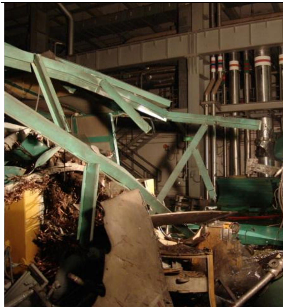
Pic#1: General View of the Generator # 7 on Slip Ring / Exciter Side
