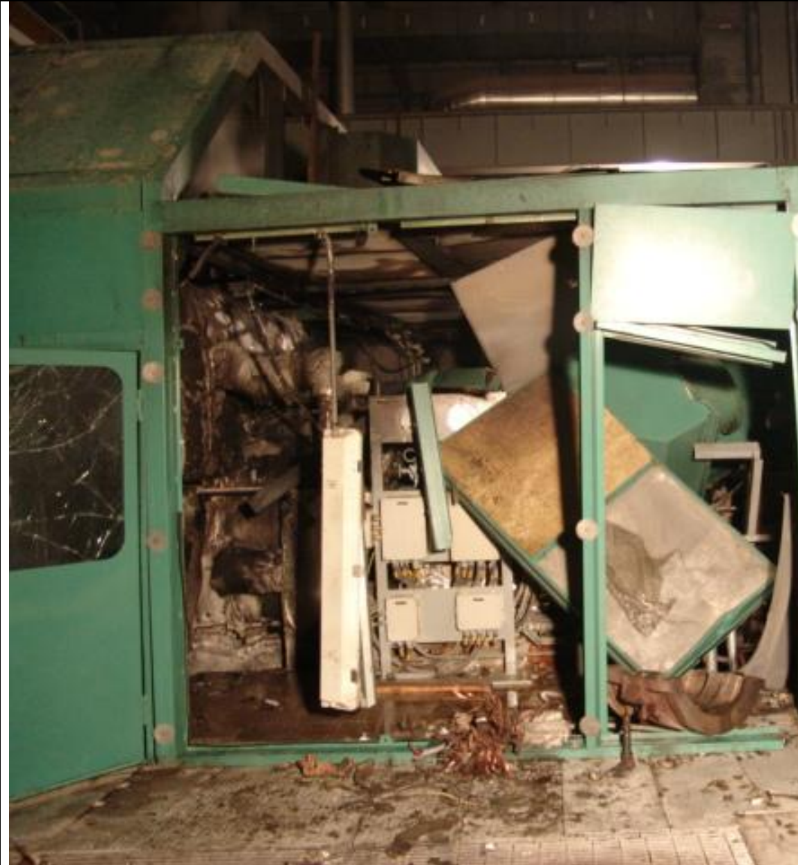
Pic# 6: Damage between Turbine-Generator Viewed from Desal Side.
