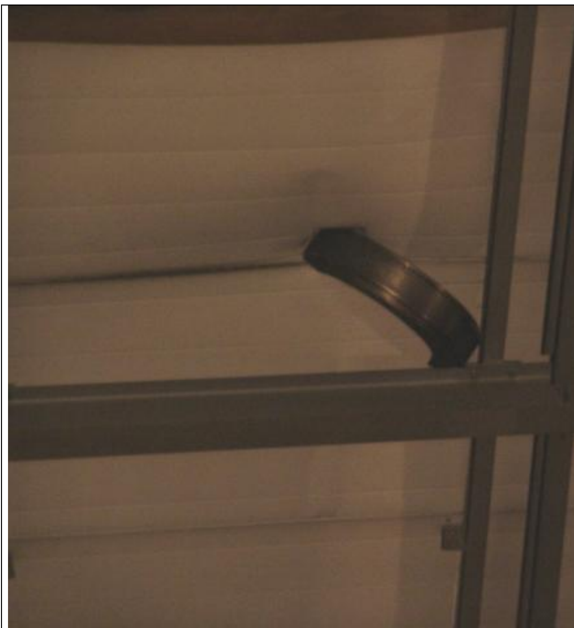
Pic# 19: A Metal Piece Flown and lying on Ceiling of the Turbine Hall.
