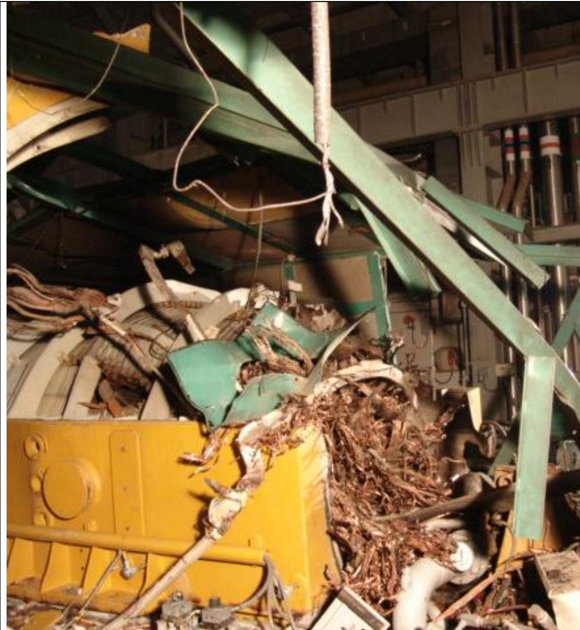
Pic#3: Extent of Damage to The Generator Viewed from Desal Side- General View.
