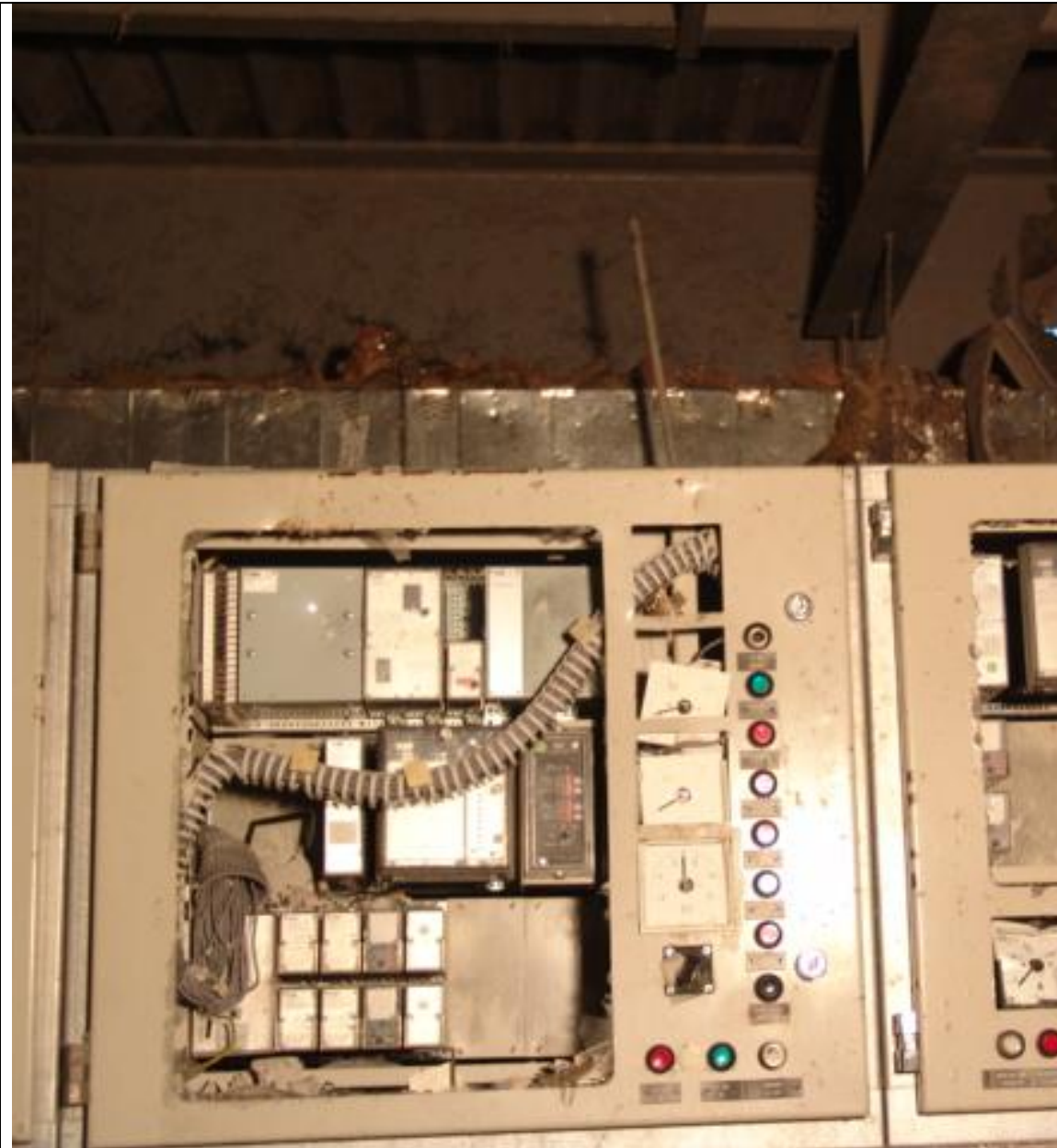
Pic# 18: Damage to Switchgears.
